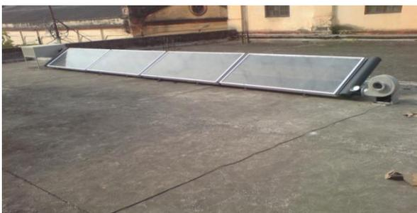
Fig. 1 Flat Plate Solar Collector [17]
