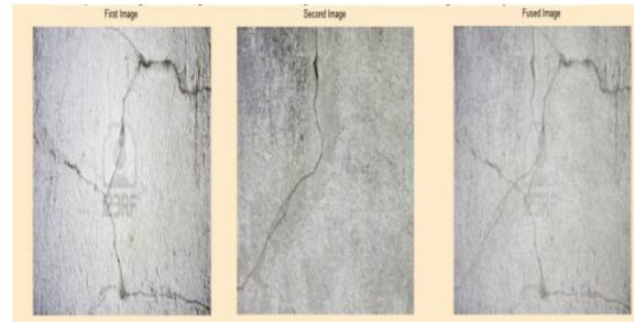
Figure 3. shows that two input image of wall cacks in same mode of initial crakes and final cracks and fused both cracks with WT technique.
