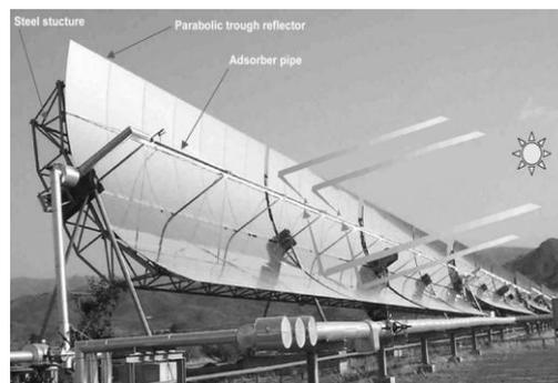
**Figure 11.** Parabolic trough collectors with steam generation system
