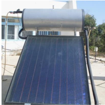
Fig.1: Passive Solar Water heating system
