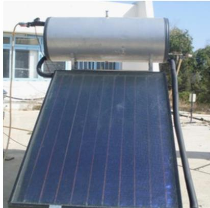
*Fig.1: Passive Solar Water heating system*
