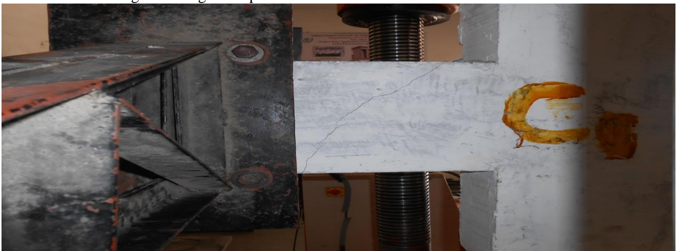
Fig.7 Controlled Beam-Column Joint No. C1 after cracking
