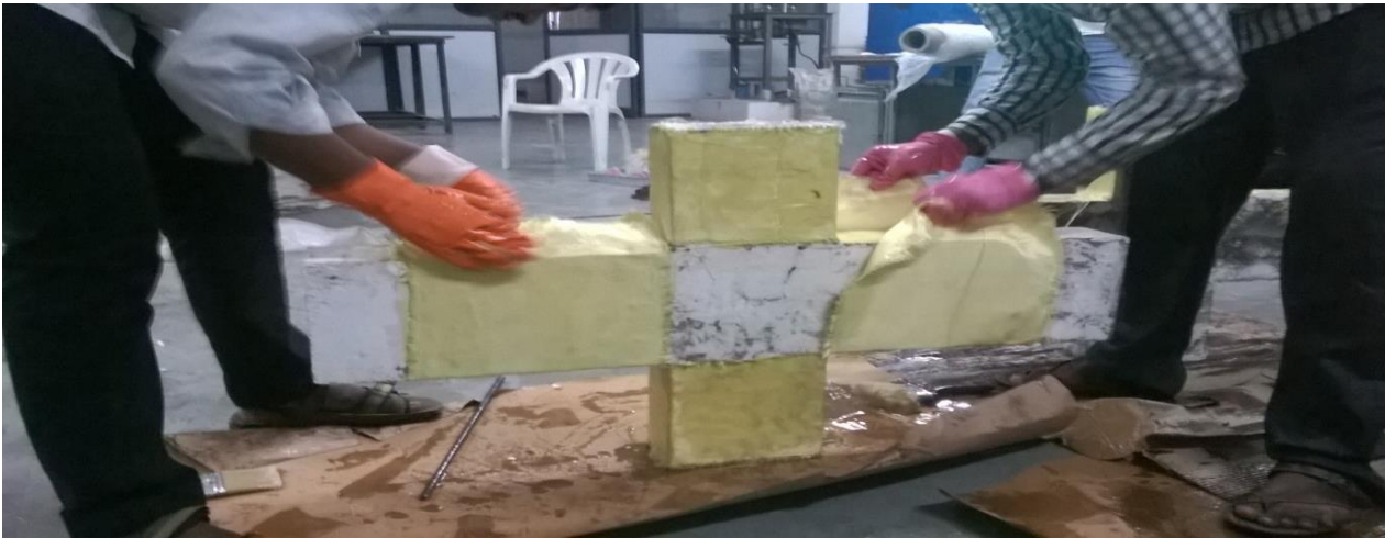
Fig.3 Fixing Aramid Sheet on Beam-Column Joint Beam-Column Joint
